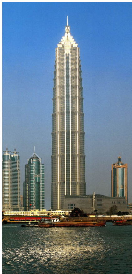
Figure 1-1: Jin Mao Tower – Shanghai, China © SOM
